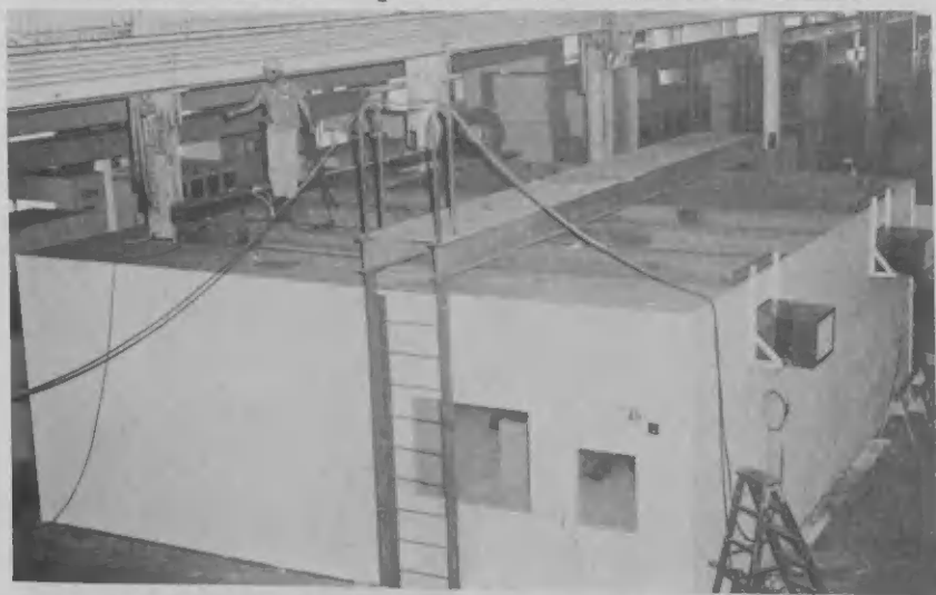
THIS NOISE-EXCLUDING office for Powerhouse No. 1 operators was designed by M. G. Murray, M. Croes and L. J. A. Halley. E OFICINA aki pa exclui zonida den Powerhouse No. 1 pa operadornan ta disenjá pa M. G. Murray, M. Croes y L. J. A. Halley.
